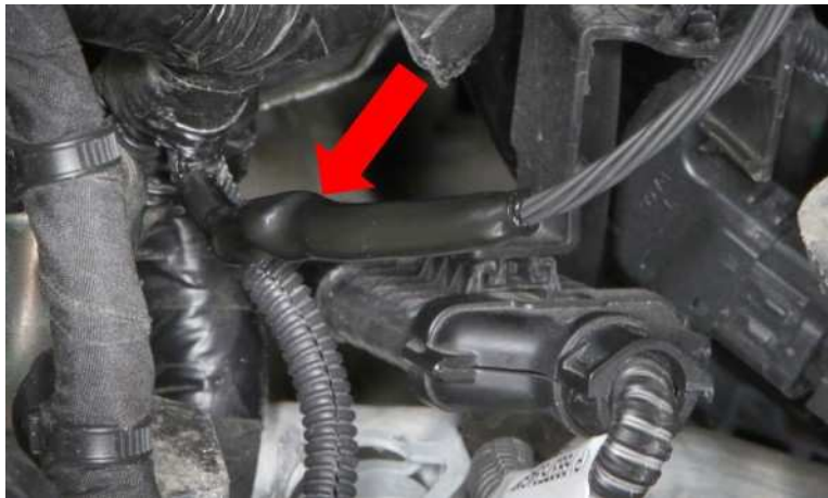
Fig. 3 Shrink Wrapped Wires
