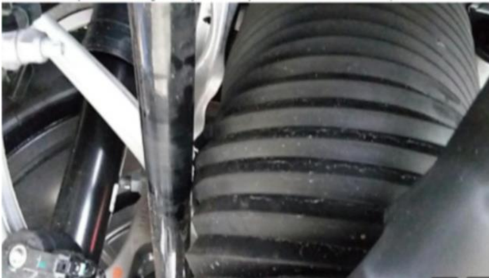
Fig 1 Bulged/bowed air spring
