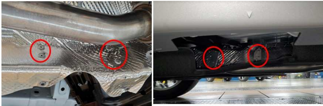
Fig. 2 Front Left Heat Shield Rivets
