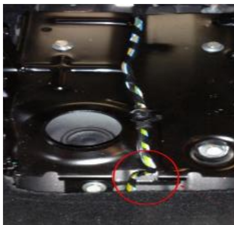
Figure 1: Point where it is possible to find a cut / interruption of the I-CAN line (white wire and blue wire)
