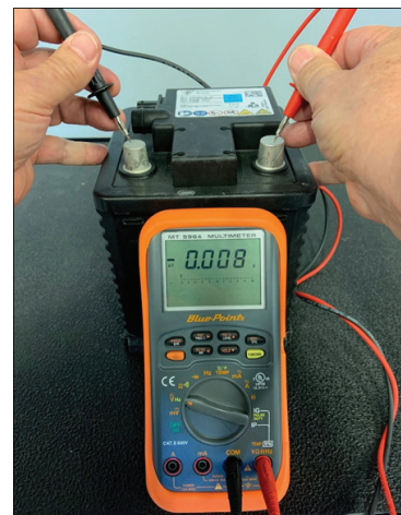
Figure 2 – Voltage test indicating an open connector
