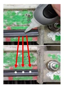
2. In addition, bond the new seal to the glass panel at the ends using adhesive P/N 07 58 9 062 157. Apply 3 small spots of adhesive at each end.
