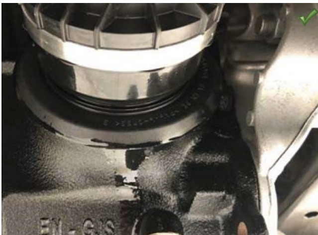
Example B: Oil is actively leaking out of the output shaft seal.
