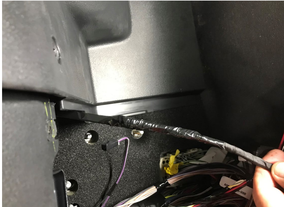
Fig. 14, End of Harness Taped to Cable Tie Inserted Through Grommet
