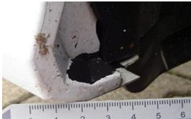
Figure 3. Interior view of the paint peel on the front lower spoiler.
