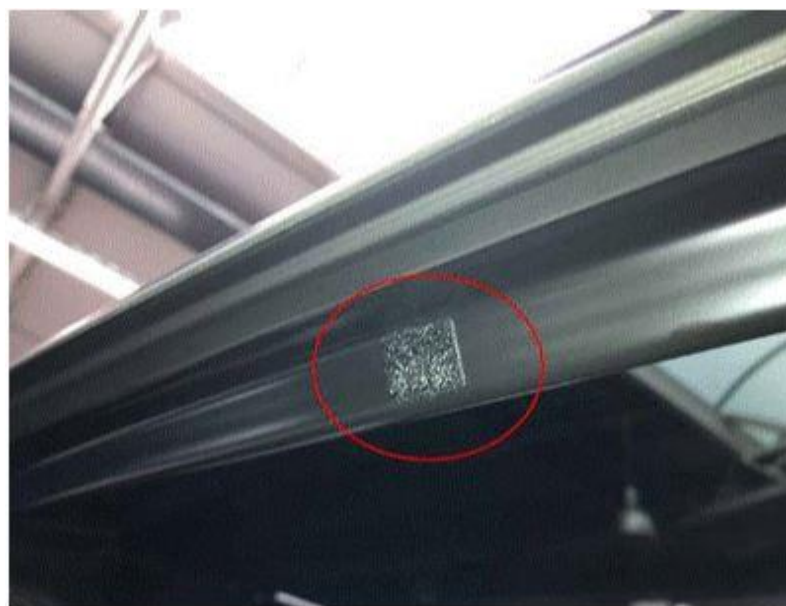
Figure 19. Adhesive felt strip material affixed to the center area of sunroof glass panel structure.
