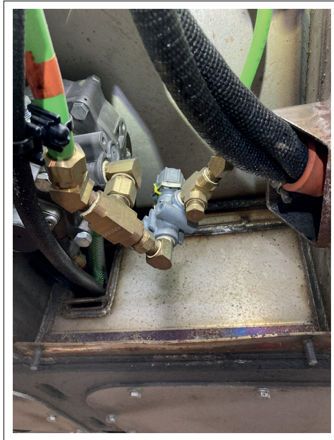
Figure 10 - Final Installation of Pressure Regulator
