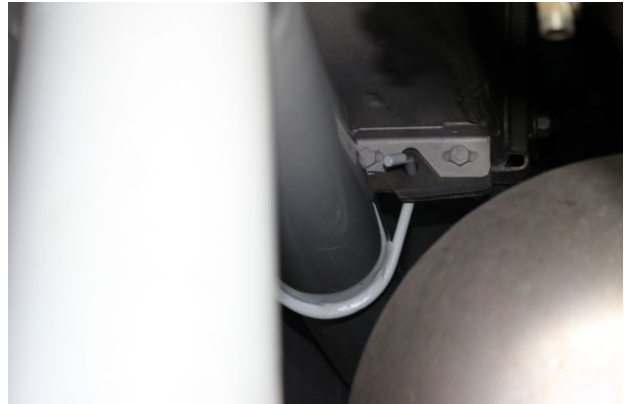
FIGURE 101: ENGINE INTAKE PIPE SUPPORT
