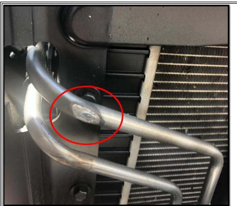
Figure #1: Inspect upper hose for signs of a rub through
