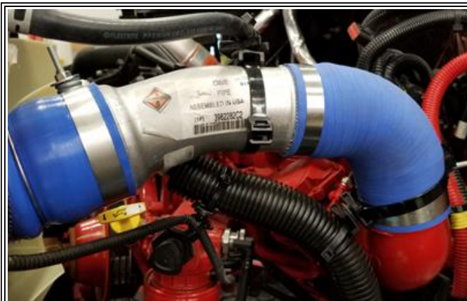
Figure 5: New CAC piping installed
