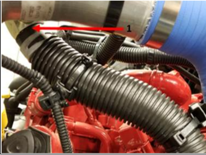
Figure 6: Air Compressor Inlet Hose
