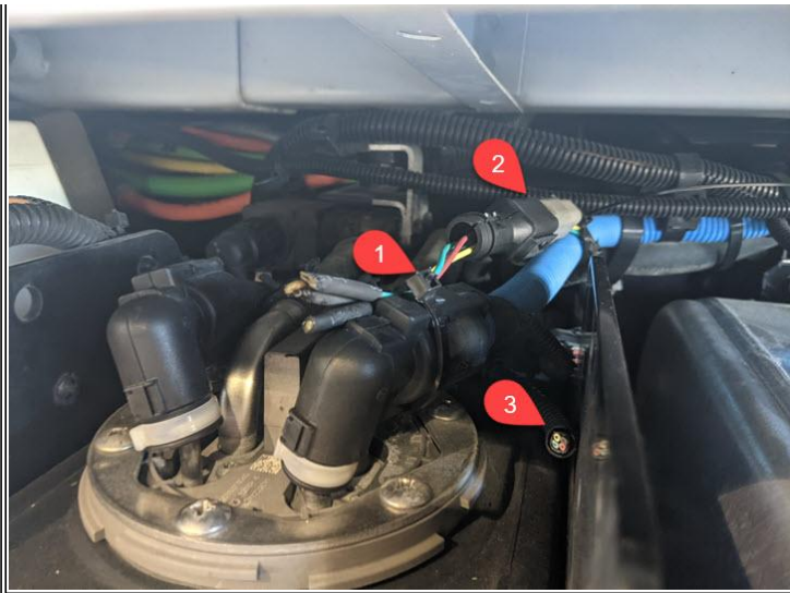
Figure 8: QLS Pigtail Installed
