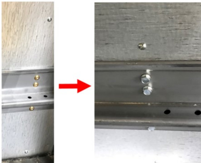
SUBSTITUTED BOLTS FOR RIVETS
