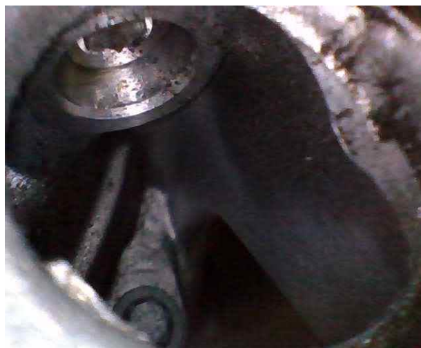
Figure 1. Missing sealing cap viewed with a pocket mirror.
