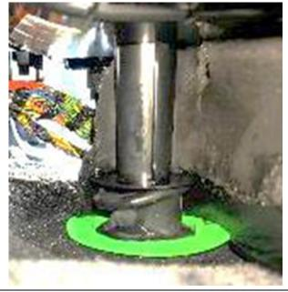
3. Here the drain hose is incorrectly installed and will require replacement to seal properly.
