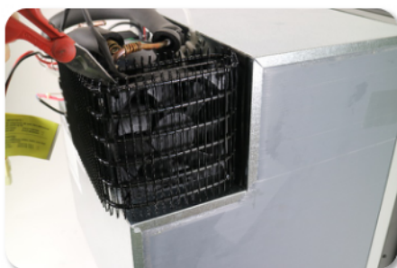
Cut the 4 zip ties fixing the fan to the condenser
