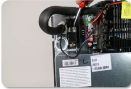
Disconnect the wires from the thermostat
