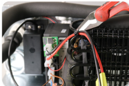
Cut the zip ties fixing the fan wires to the condenser
