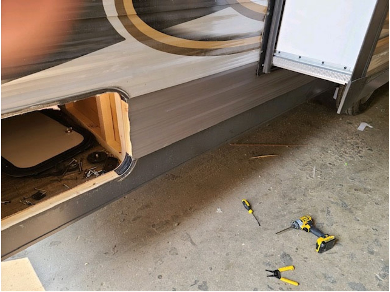
Slide out repairment final look
