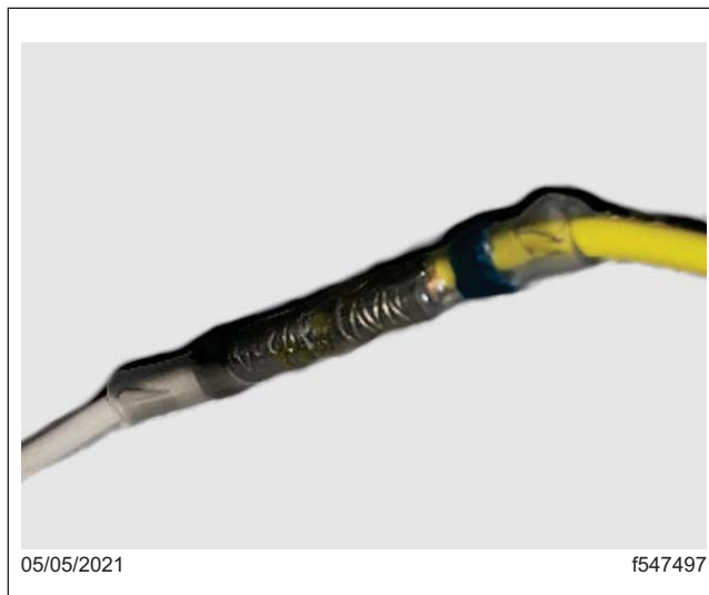
Fig. 13, Incorrectly Sealed Solder Sleeve
