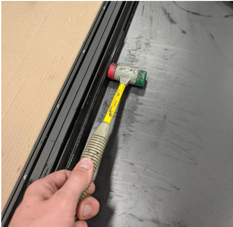
Figure 9: Install Continuous Window Channel Cover
