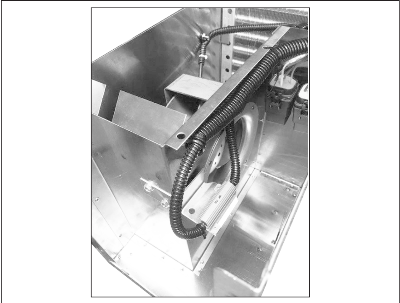
Figure 8 - Installation of the New Bundle
