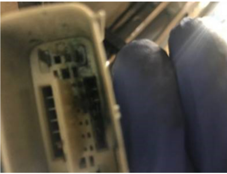
Example of damaged connector at plugged cavity, which may displace the cavity plug, allowing water to enter.
