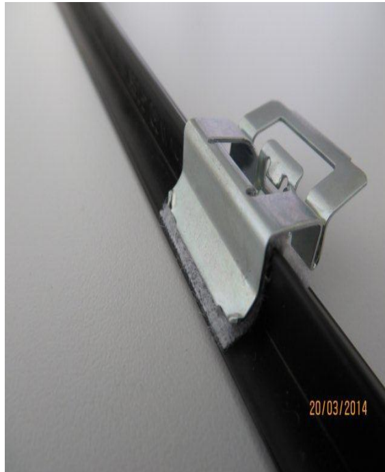
Figure 4. Retaining clip isolated with the fleece adhesive tape.
