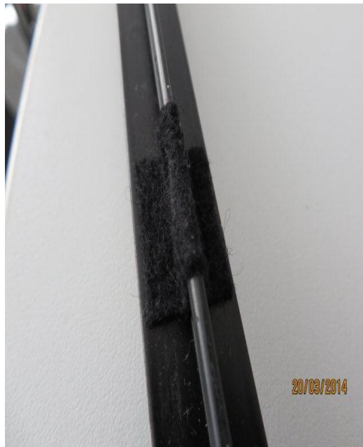
Figure 3. Fleece adhesive tape section applied.
