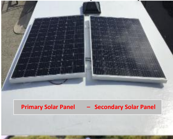
FIG - 1 Solar Panels – Primary and Secondary Panels
