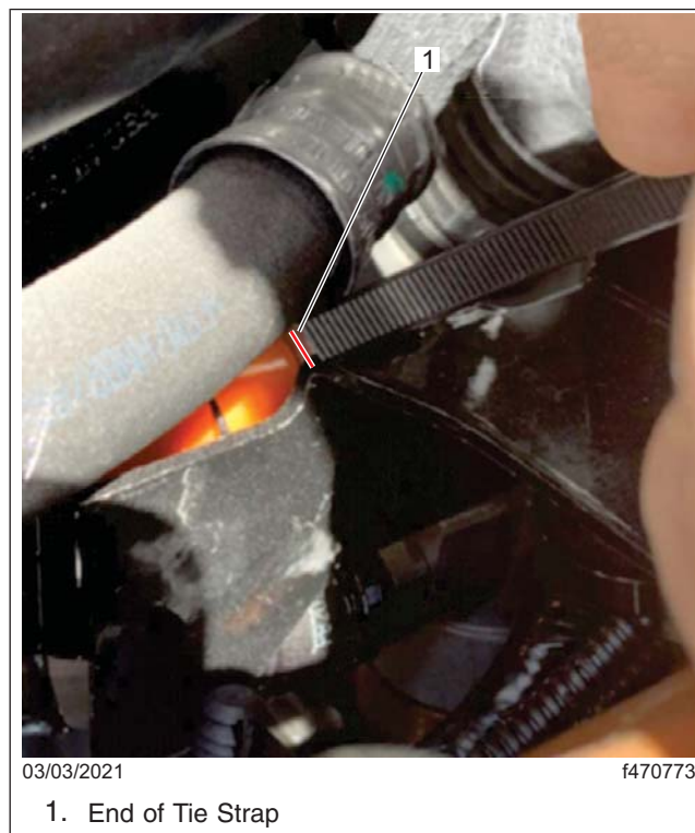
Fig. 3, Measuring Fuel Line Clearance
