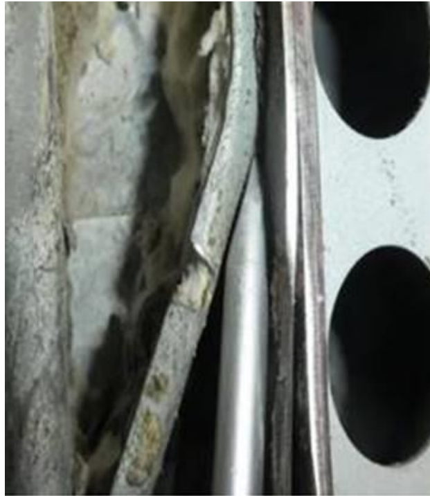
Figure 23. The chisel end of the steel rod properly engaged with the reinforcement plate.
