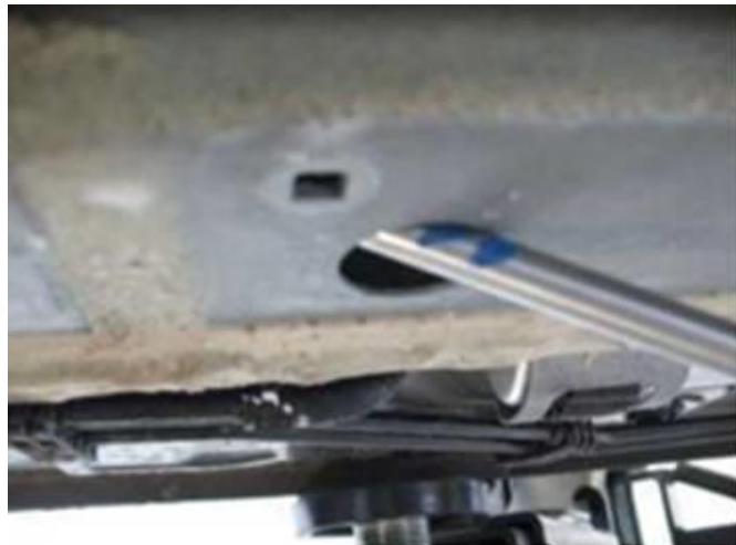
Figure 25. Marking the steel rod.
