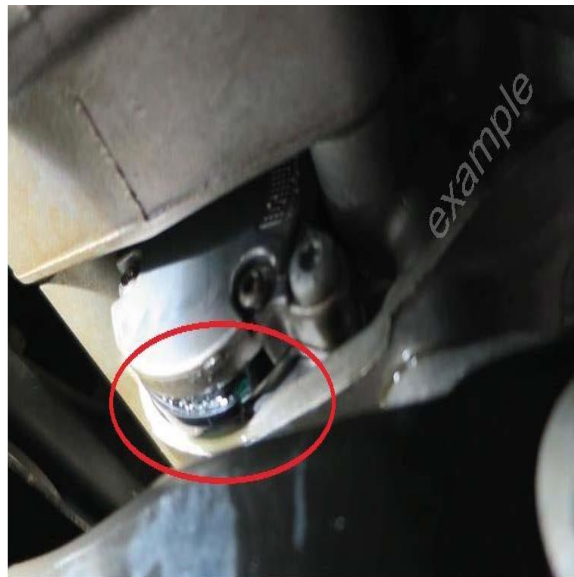
Figure 1. Oil leaking in area of the auxiliary hydraulic pump (V475).
