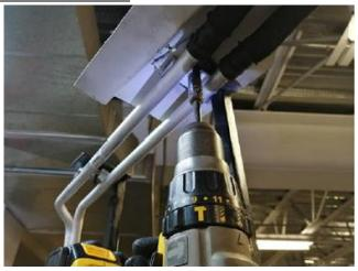
1. Loosen and slightly lower the underfloor coolant pipe in the affected connection area.
