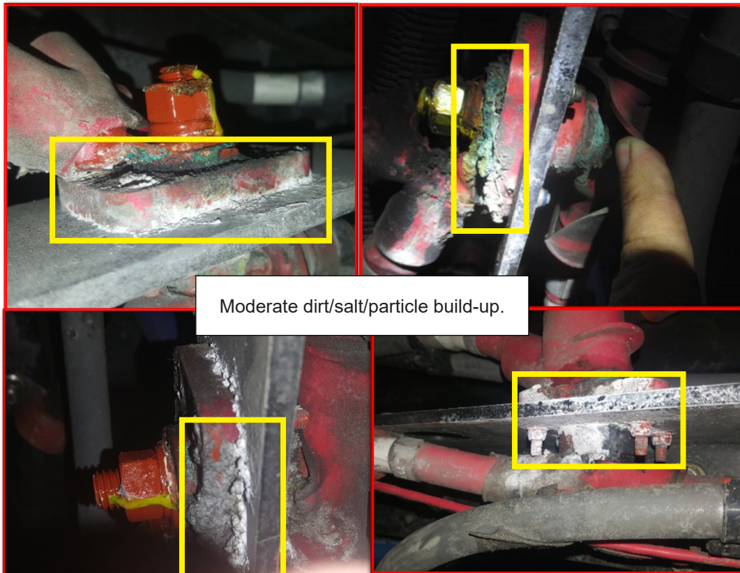
Figure 7 - Need of Maintenance for Junction Blocks with DOLPH ER-41/EB-41 Corrosion Preventative Product
