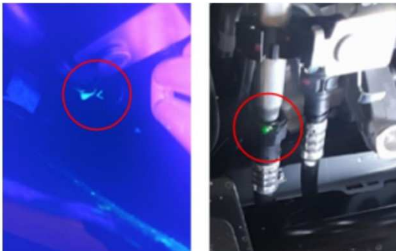
Fig. 1 Areas To Check For Leaks
