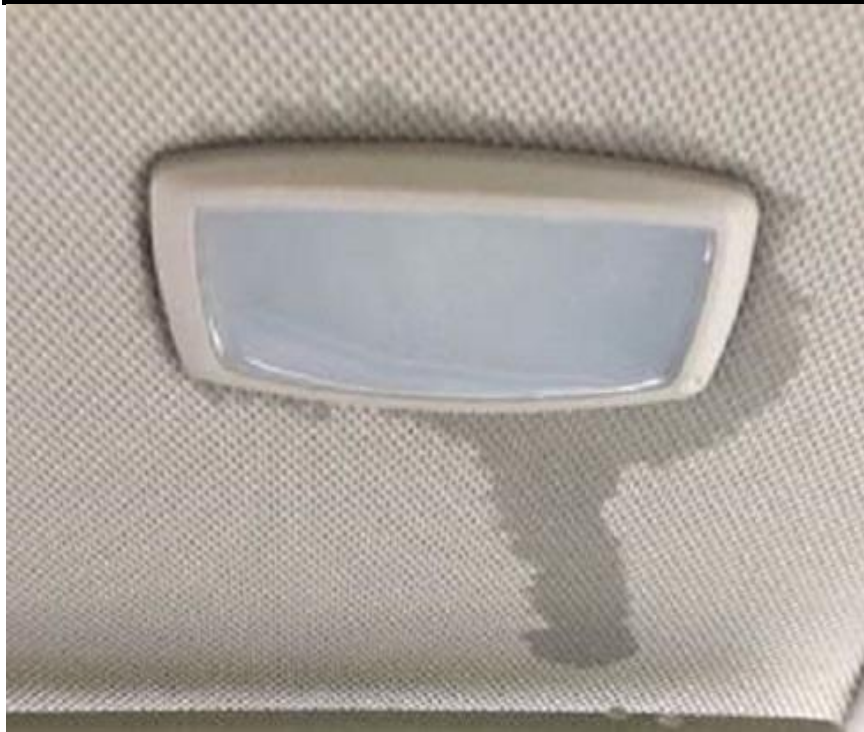
Figure 1: Example of water leak coming from the front vanity light.
