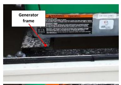
2. Center the close-off angle with the pre-drilled screw holes on the top of the generator frame. The (side) of angle should be directed down and against the door frame.
