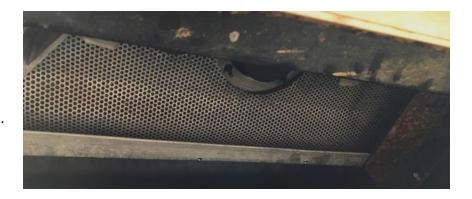
3. Place the front of the plenum against the sidewall of the unit. Install (2) self-tapping screws on each end of the plenum in the pre-drilled holes. Install (4) self-tapping screws in the pre-drilled holes on the back of the plenum.
