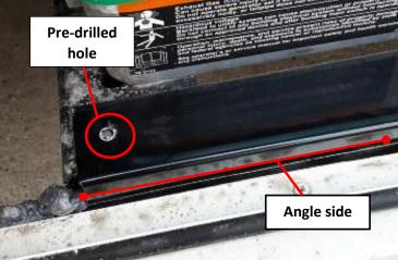
3. Install (1) self-tapping screw at each end of the angle in the pre-drilled hole.
