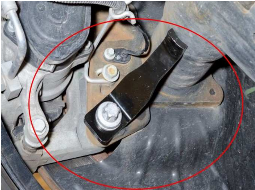
Fig. 2 One Bracket Installed into Position
