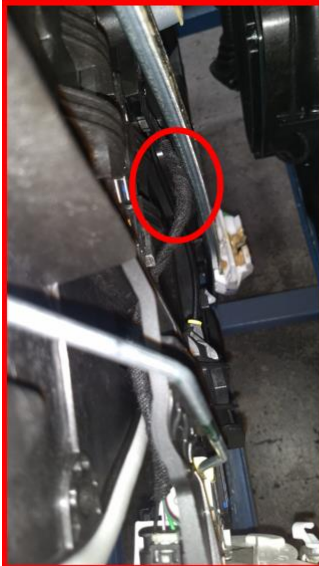
Top Down View Of Harness Making Contact With Rear Window Rail (Door Carrier Plate Removed)
