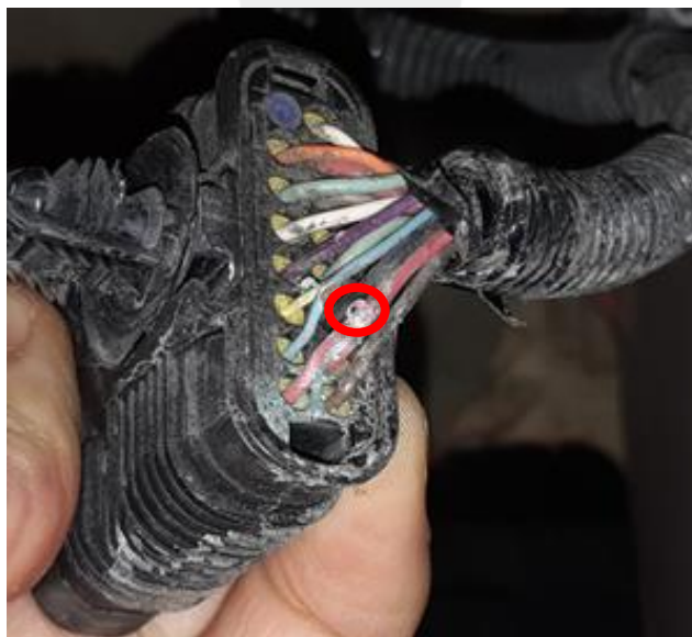
Figure 6 – Damaged electrical circuit at X952
