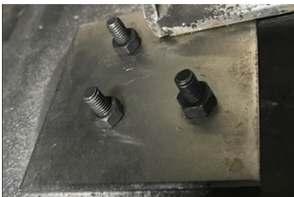
FIGURE 22: REINFORCEMENT PLATE INSTALLED
