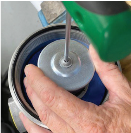
Figure 8 - Steel Cap Installation
