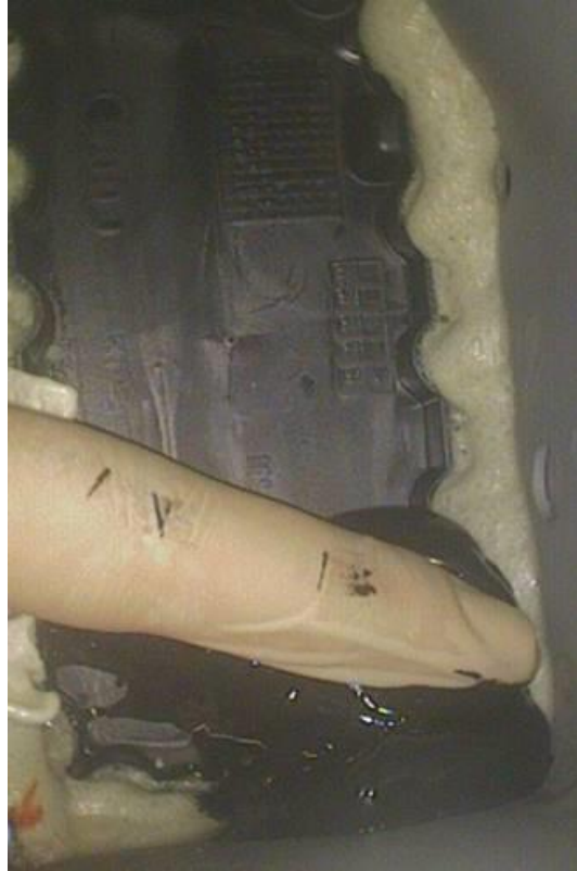
Figure 10. Distributing sealer over the web plate.
