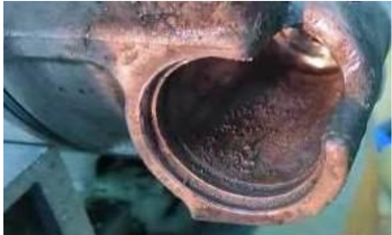
Figure 10. Corrosion in the N280 valve bore.
