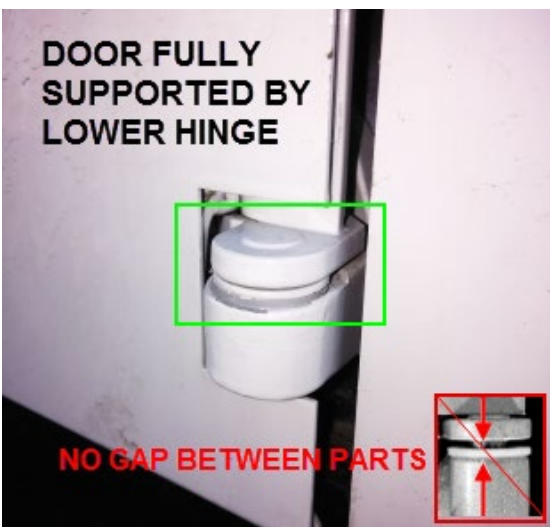
FIGURE 7: LOWER HINGE SUPPORT
