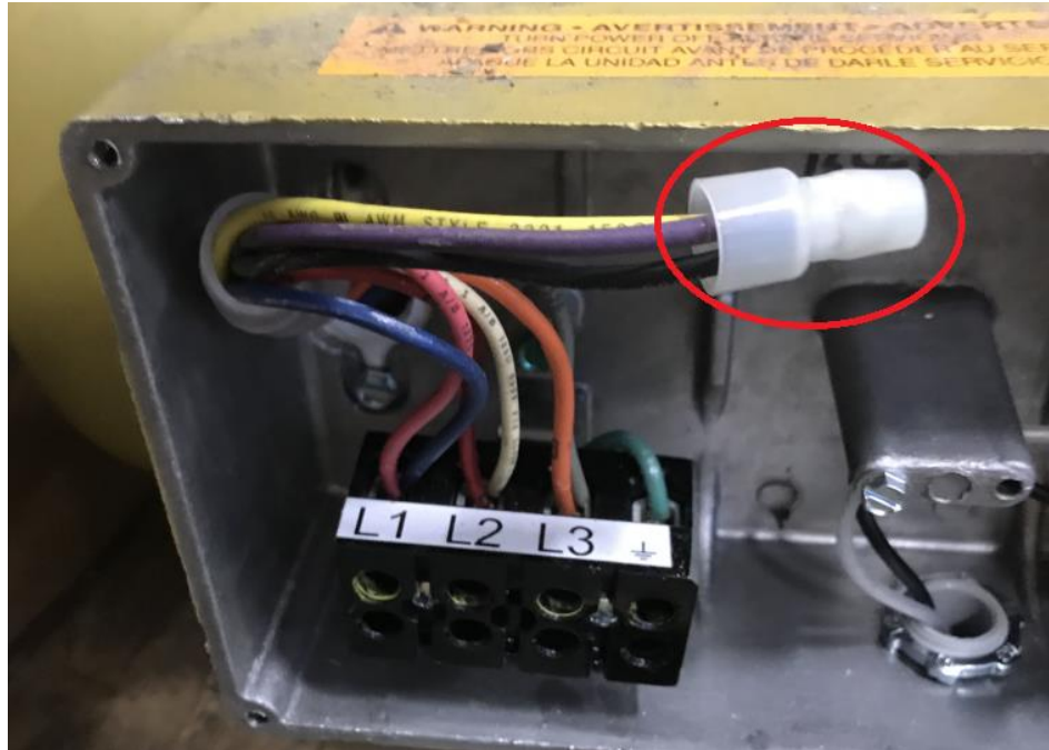
Figure 3: Closed End Crimped Splice
