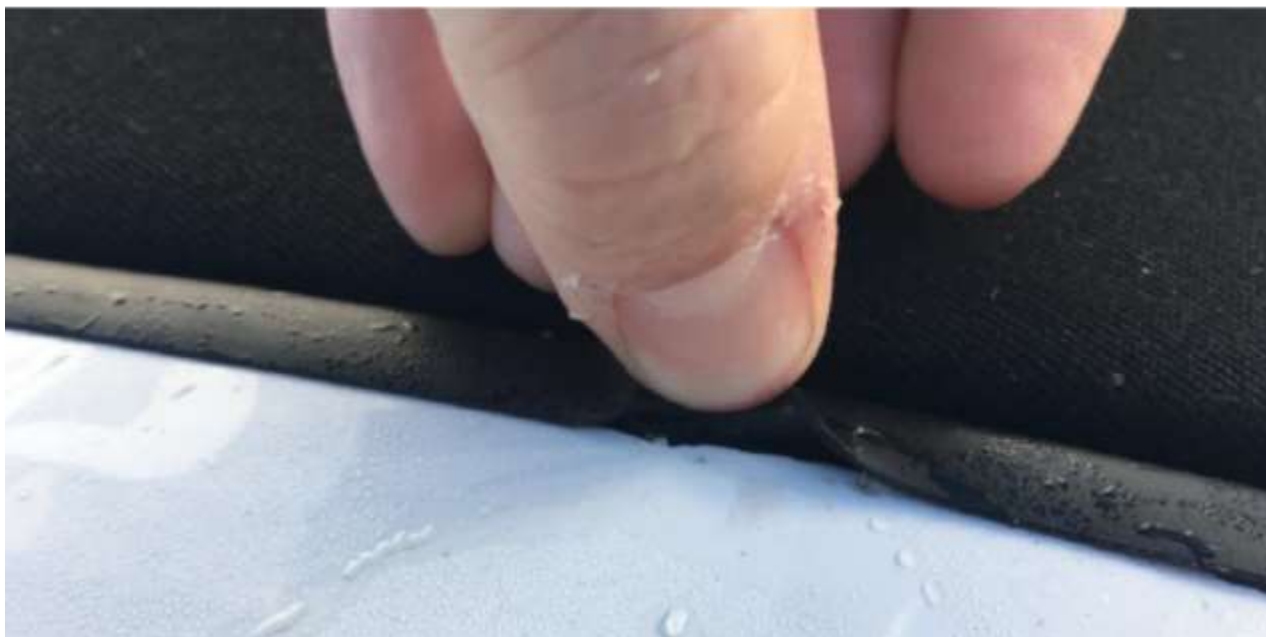
Fig 3 inspect for butyl void(s).
