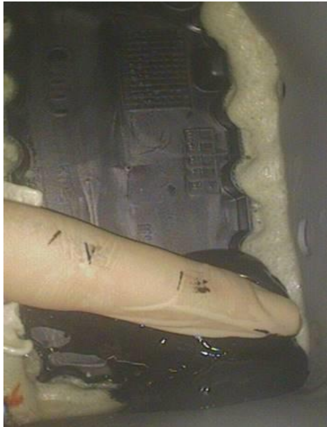
Figure 10. Distributing sealer over the web plate.
