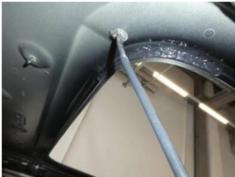
Figure 11. Filling the cavity with foam.
