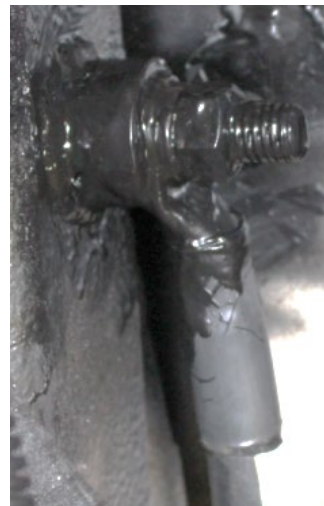
FIGURE 126: GROUND STUD WITH RUBBER COATING
