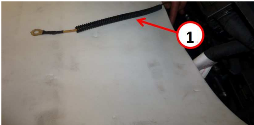
Fig. 8 Wire Inside Corrugated Sheath
