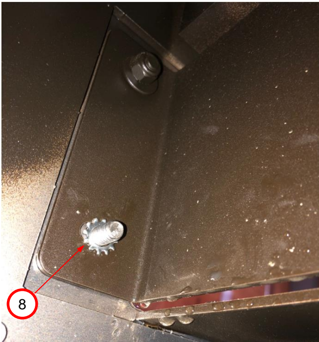
Figure 4: Star washer installed (8)
