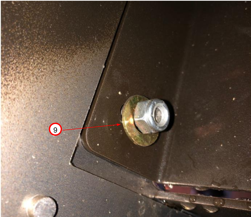
Figure 5: Flat washer and nut reinstalled (9)
